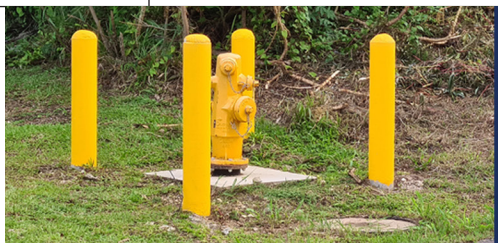
Installation of a New Fire Hydrant
