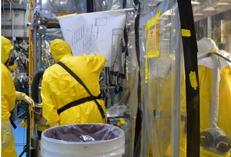
Equipment removal in the Plutonium Facility at LANL.
