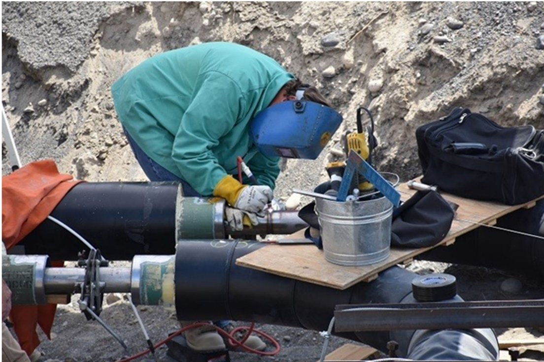
Worker installing a transfer line that will transport waste between facilities at Hanford.
