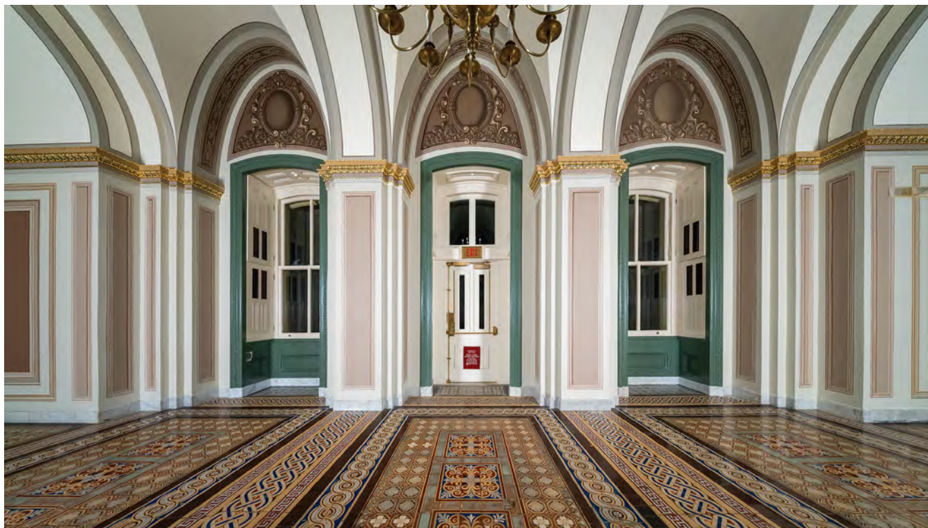
The Senate Connecting Corridor on the first floor of the U.S. Capitol following plaster repairs and painting to replicate historic design elements.
