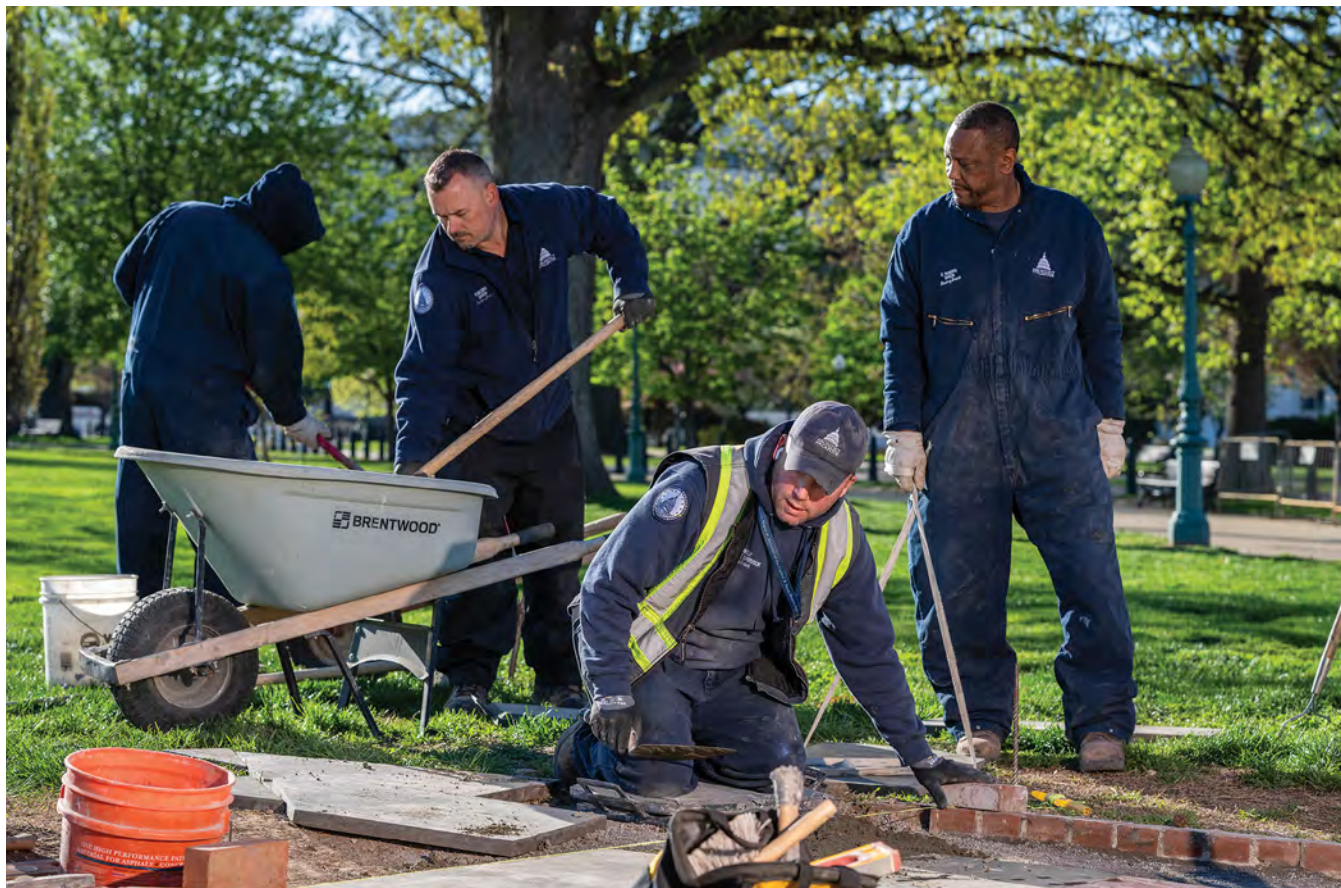
Stone pavers are repaired on the East Plaza of the U.S. Capitol.
