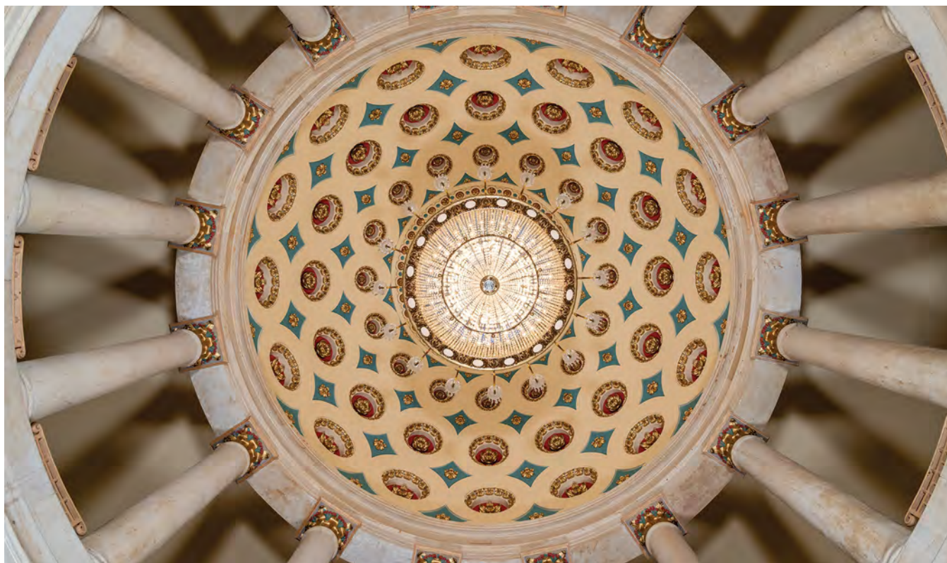
Ceiling of the Small Senate Rotunda in the U.S. Capitol, featuring restored decorative detailing and lighting.
