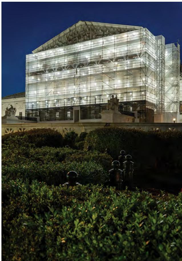
The west façade of the Supreme Court of the United States illuminated at night, with scaffolding in place for exterior restoration work.
