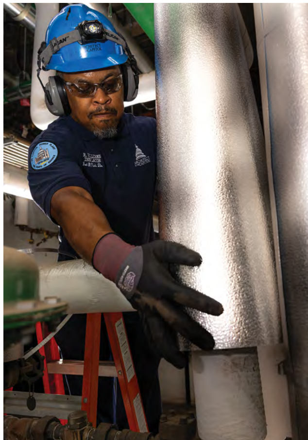
Insulation is installed at the Capitol Power Plant to improve energy efficiency and system performance.
