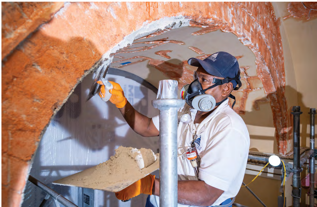
Plaster repairs in the first floor Senate Connecting Corridor of the U.S. Capitol help preserve the historic vaulted ceiling.
