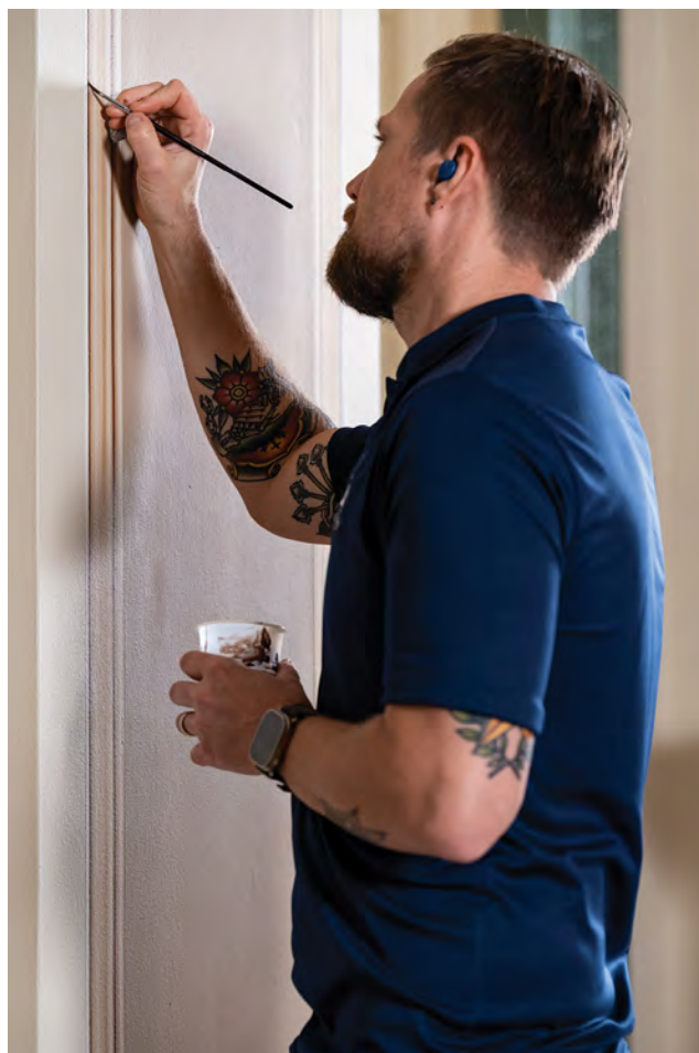
Plaster repairs and trompe-l'œil detailing in the Senate Connecting Corridor of the U.S. Capitol.
