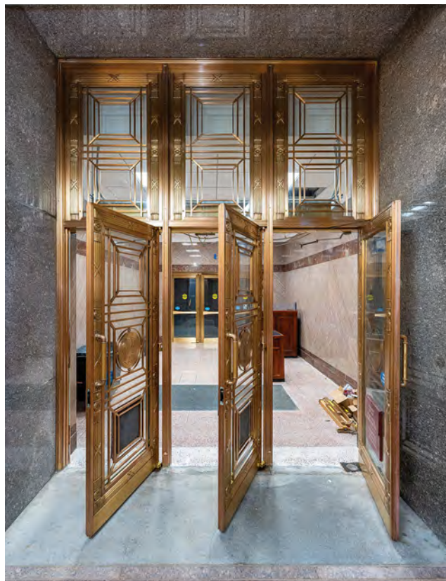
Bronze doors in the Dirksen Senate Office Building are included in a broader effort to conserve the building's historic entrances.
