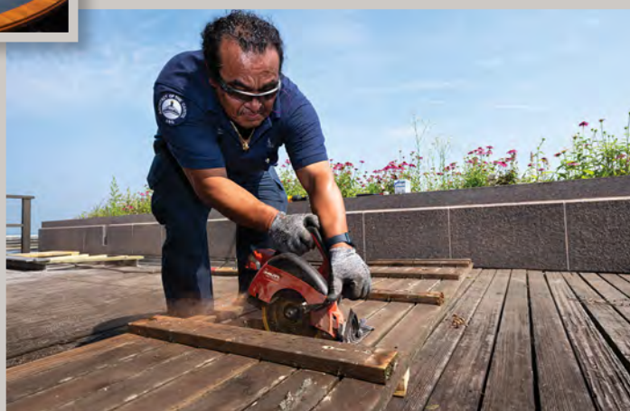
Decking is replaced on the sixth-floor terrace of the James Madison Building.
