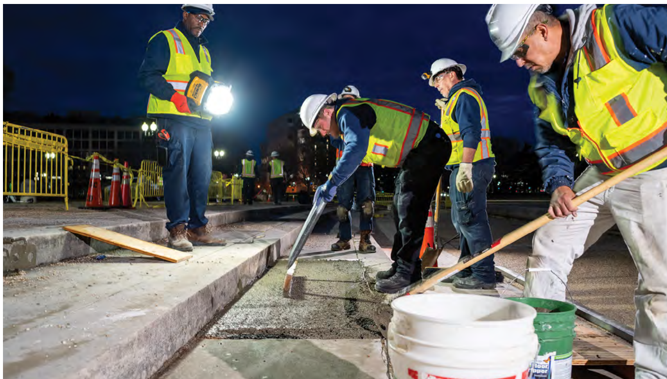
Steps are repaired at the Capitol Reflecting Pool in front of the U.S. Capitol.
