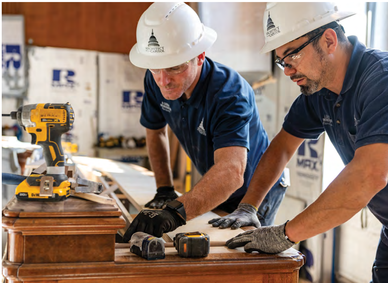
Carpentry work underway as part of ongoing construction and renovation activities at the Dirksen Senate Office Building.
