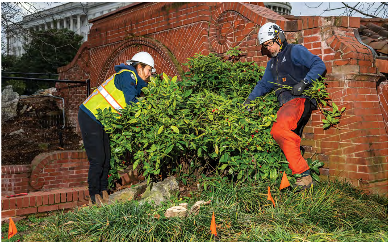
Landscape restoration work at the historic Olmsted Summerhouse on the U.S. Capitol Grounds.
